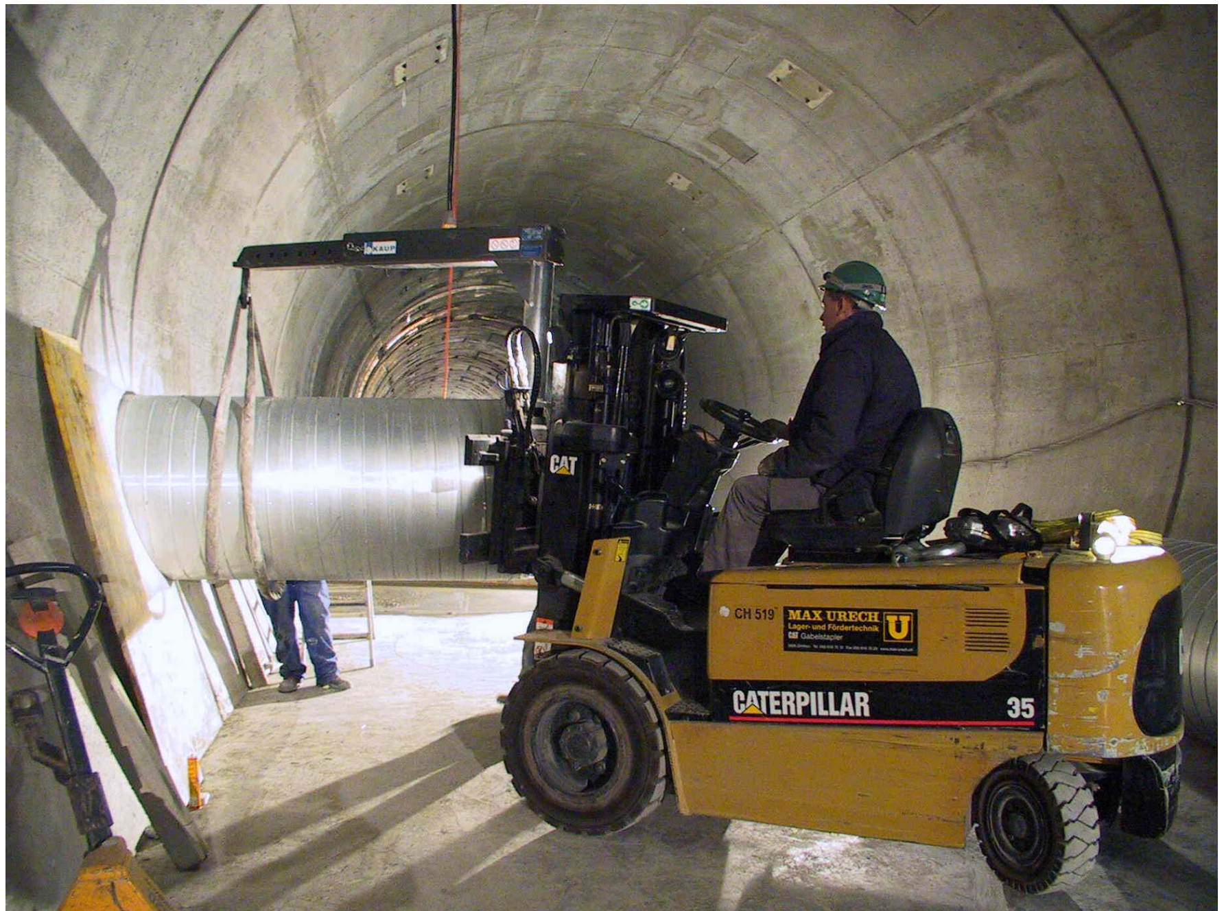
Installation of Steel Duct in Target Chamber (11/10/2004)
