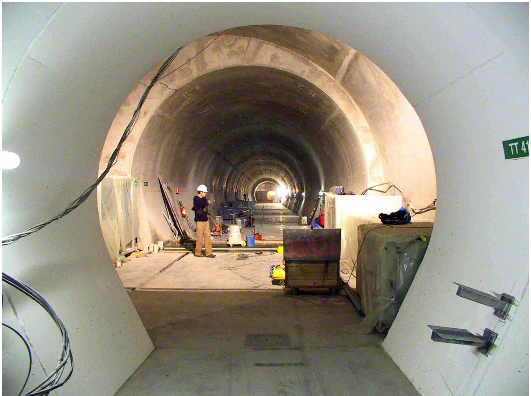
View of Target & Junction Chambers from Proton Beam Tunnel (28/10/04)
