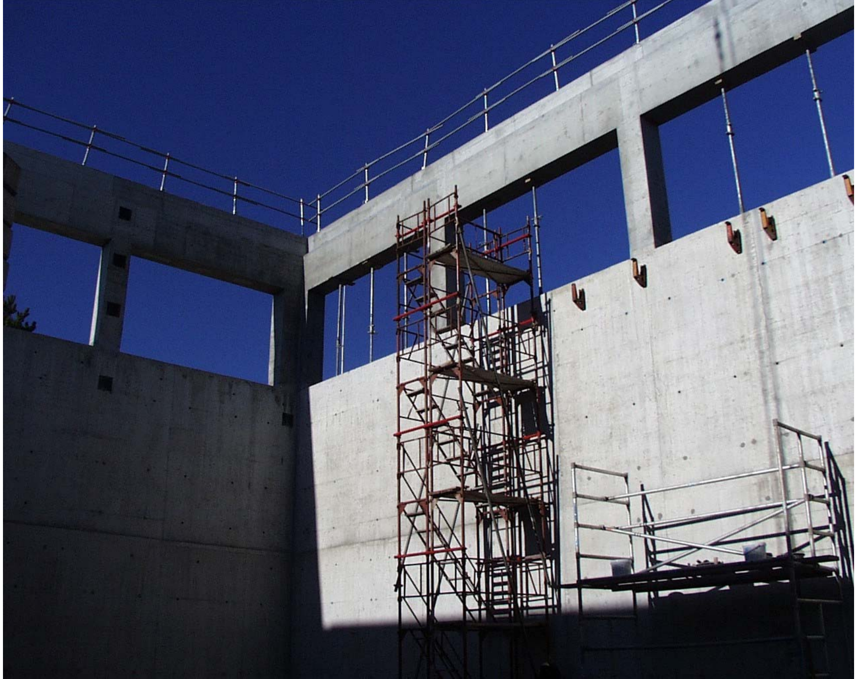
View of Building 170 (15/11/04)
